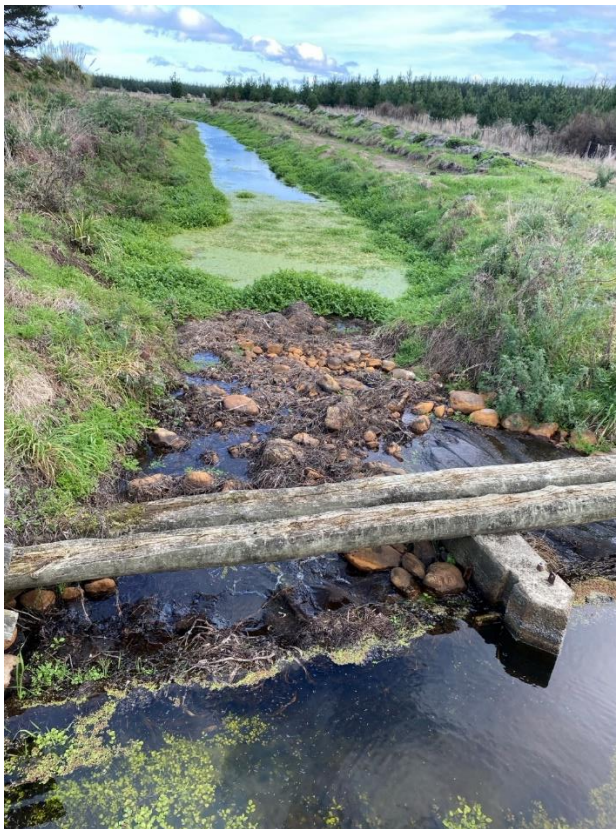
Figure 17: Fish Pass and section of perimeter outlet on private property
